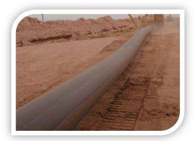
DRISCOPLEX® 9200 Series Liner Pipe is used in pressure applications as an HDPE liner for existing pipelines. The dimensions and tolerances are customer defined for each specific application.
